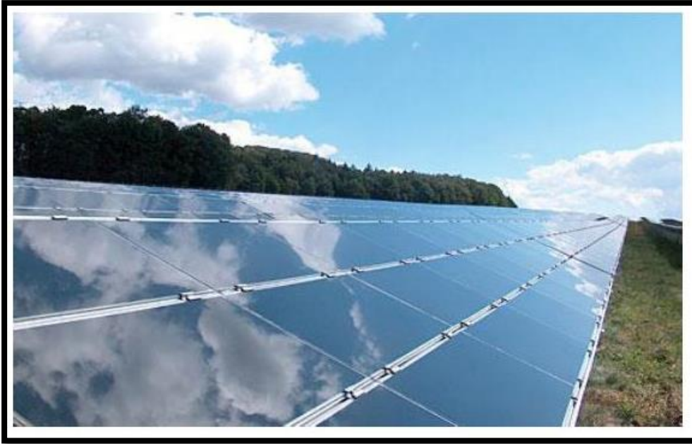
Figure I.18: Cadmium Telluride glass-glass modules, efficiency of 9 to 11%. [17]
